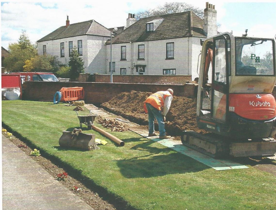
Pl. 73 Service trench, looking south-east towards churchyard south wall.
