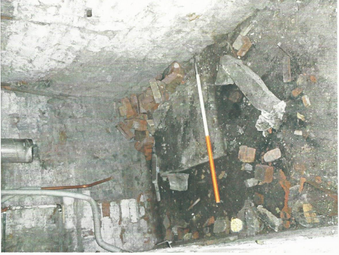
Pl. 54 Tower boiler cavity after removal of the boiler, looking north-west. Scale 1m.
