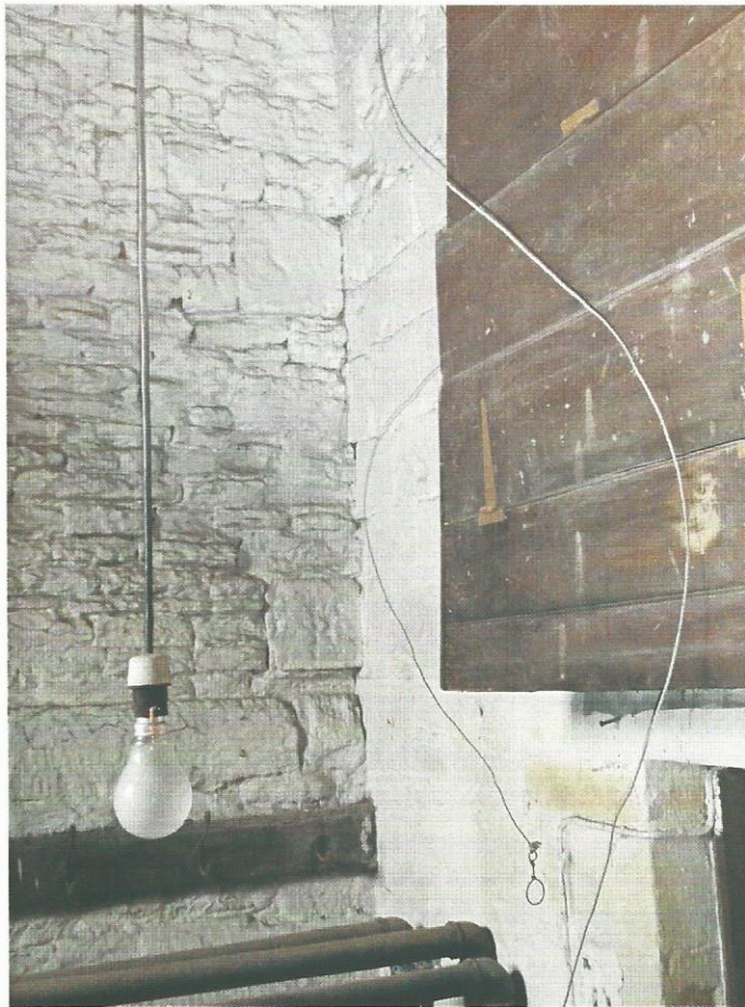
Pl. 61 Junction of the tower north wall with the earlier nave west wall, showing the contrast of ashlar blocks in the nave wall with the roughly dressed stonework of the tower wall.
