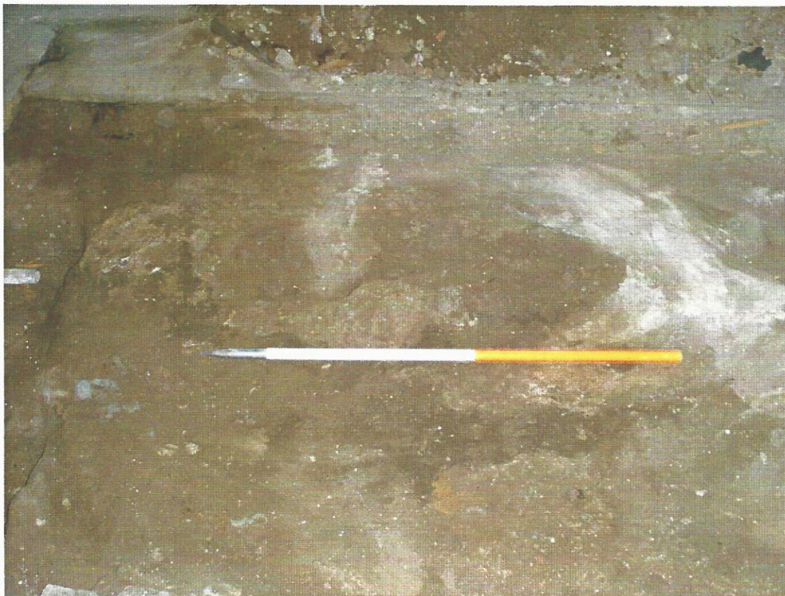
Pl. 18 Mortar patch 206, looking south. Scale 1m
