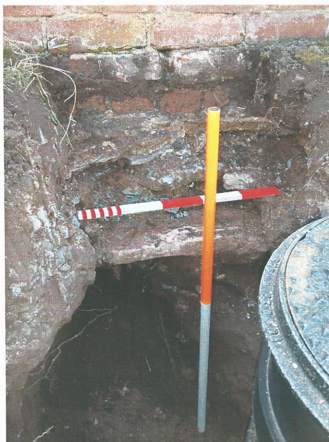
Pl. 74 Churchyard, south boundary wall external face next to new manhole, looking north. Scales 1m and 0.50m
