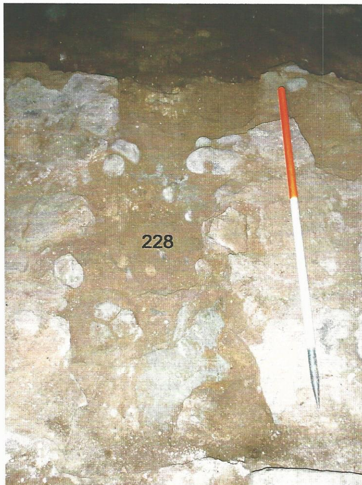
Pl. 14 Damaged area of wall 201 for pew support, with posthole 228 beneath, looking south. Scale 1m
