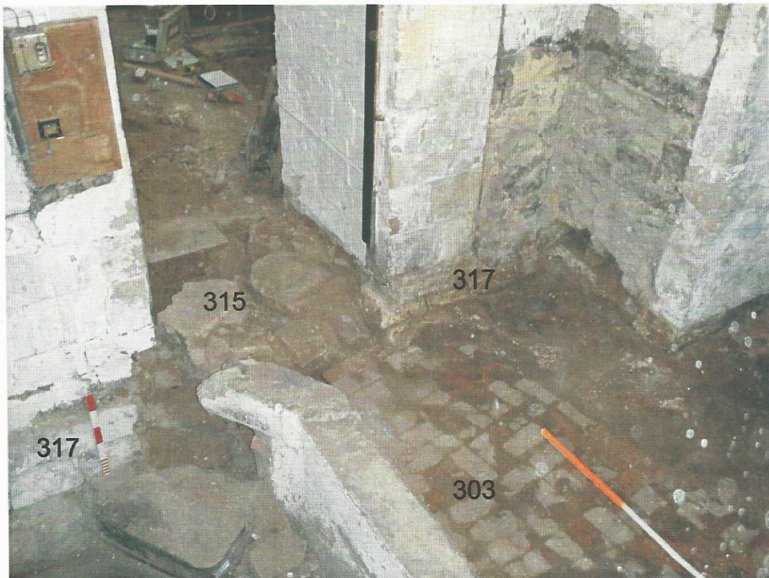
Pl. 64 Tower door threshold after removal of concrete steps, looking south-east. Scales 1 and 0.50m
